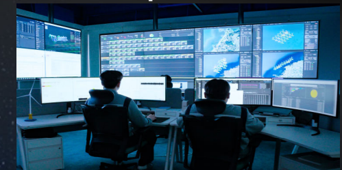
Advanced O&M (Wind Power Center)
